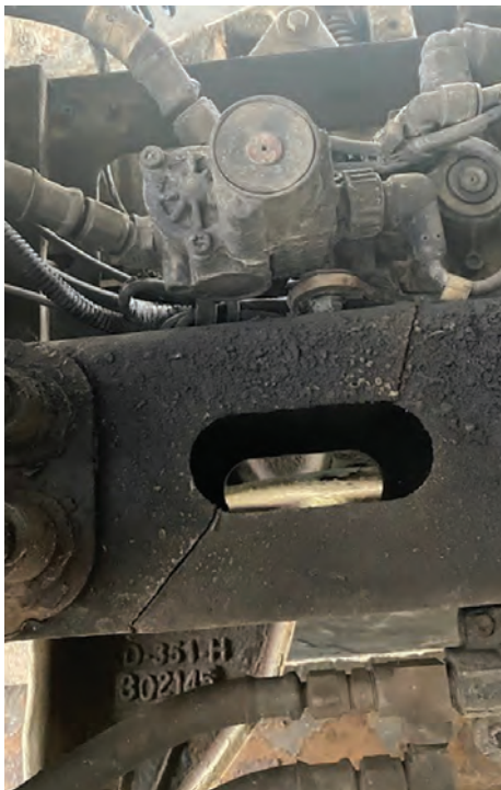
Submitted by Cpl. Gustavson: Cracked frame crossmember on a truck.
